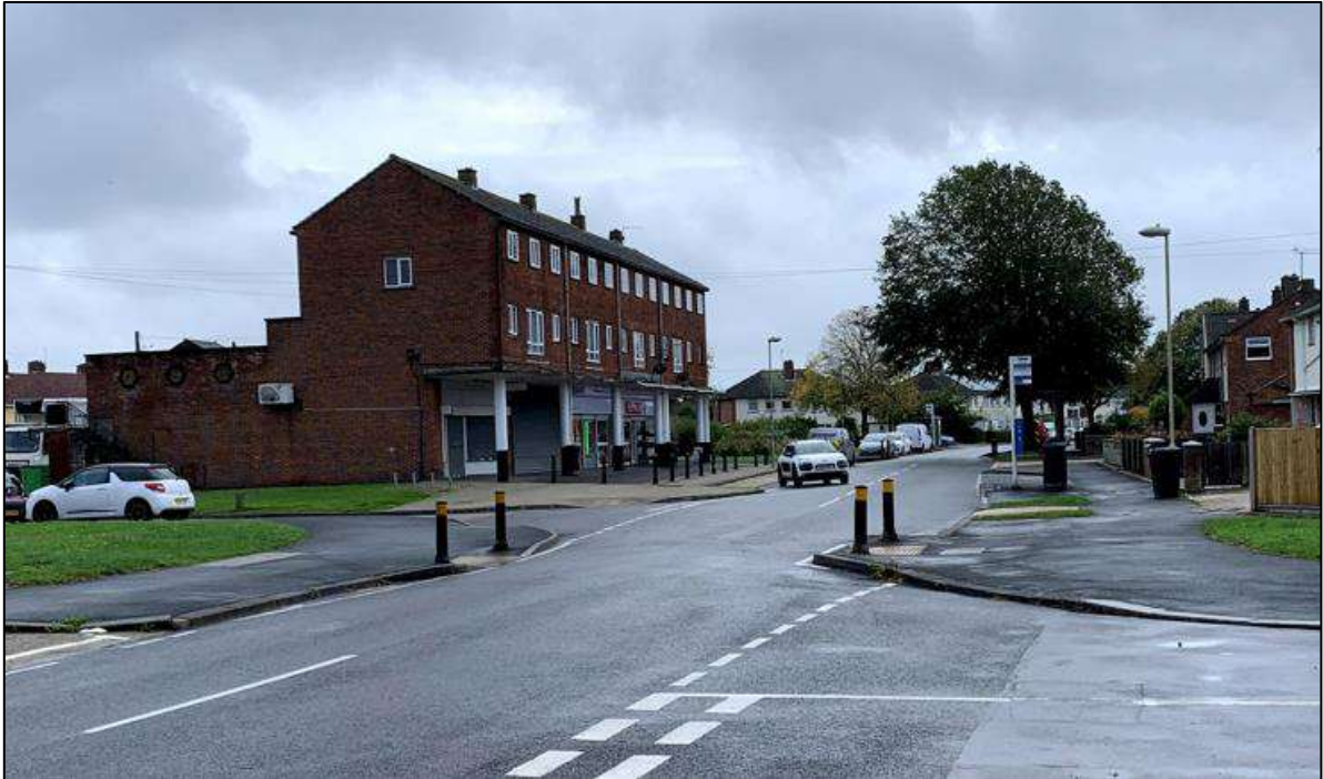
Image 13: Crossing Facilities Adjacent to the Tukes Avenue Local Centre
