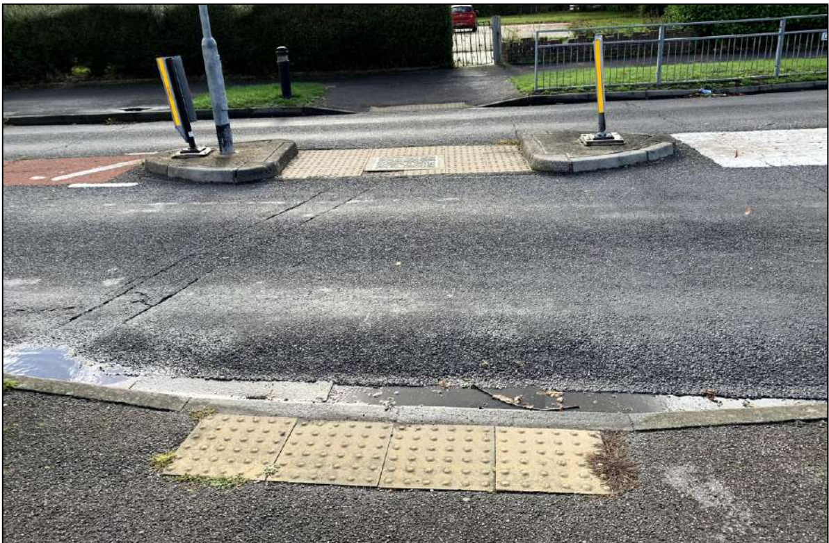
Image 14: Dropped Kerb with Tactile Paving Crossing Across Gregson Avenue
