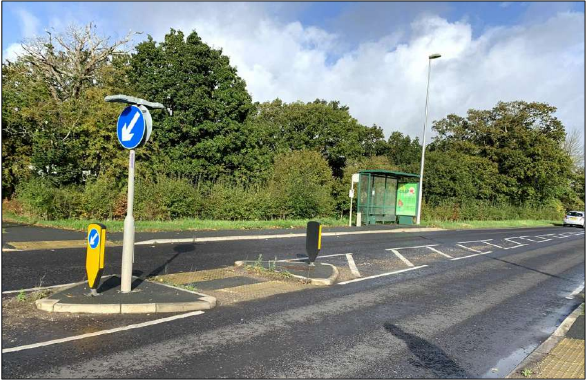
Image 18: Refuge Island crossing across Newgate Lane East
