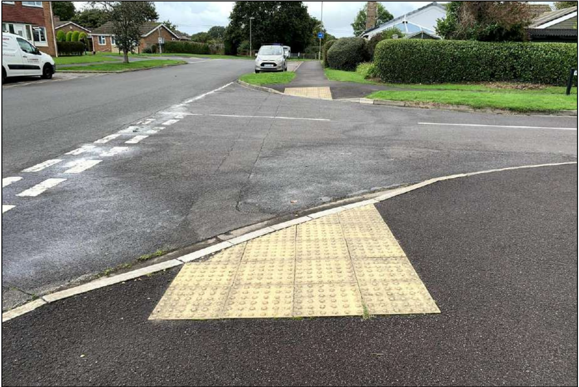
Image 9: Dropped Kerb Crossing with Tactile Paving Along Brookers Lane
