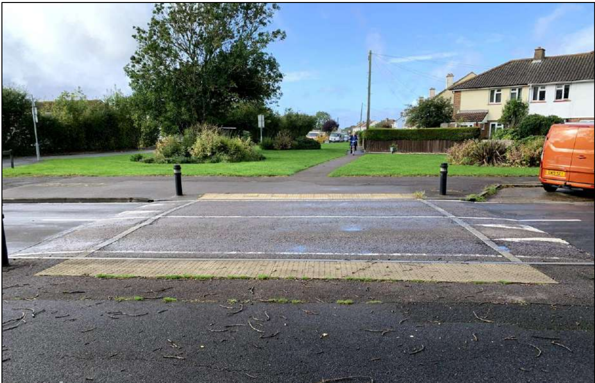
Image 10: Dropped Kerb Crossing with Tactile Paving on Wych Lane at Holbrook School
