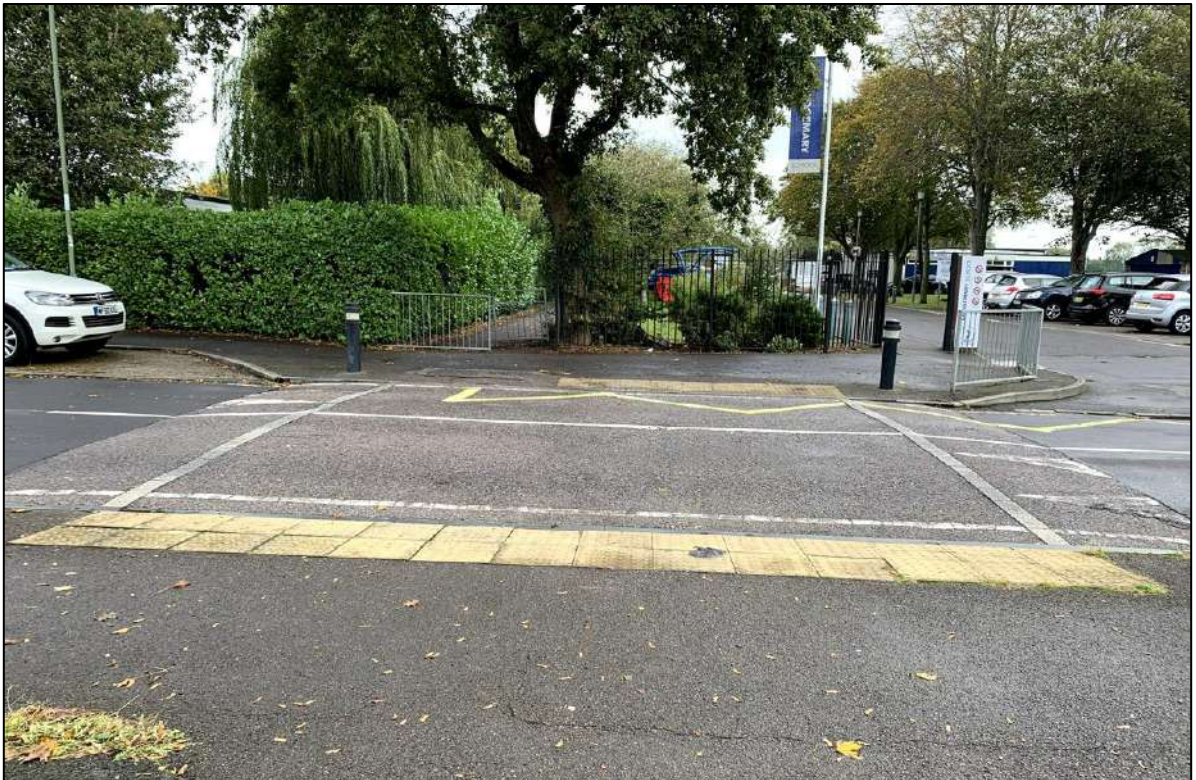
Image 12: Dropped Kerb Crossing with Tactile Paving on Wych Lane at Bridgemary School
