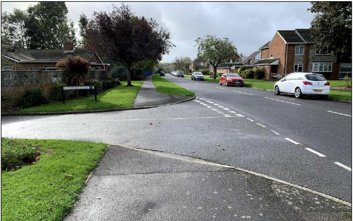
Image 3: Dropped Kerb Crossing Across Kittiwake Close along The Drive
